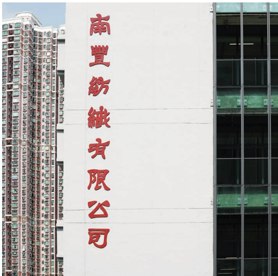
外牆的“南豐紡織有限公司”字樣在修復過程重新倒模，並堅持沿用式微工藝重新製作及置於原位，寓意“ The Mills ”承先啟後。The characters “南豐紡織有限公司” on the façade were re-moulded during renovation. Re-made with the same micro-process as before, they remain in their original place, implying that “ The Mills ” will uphold the past and shape the future.
