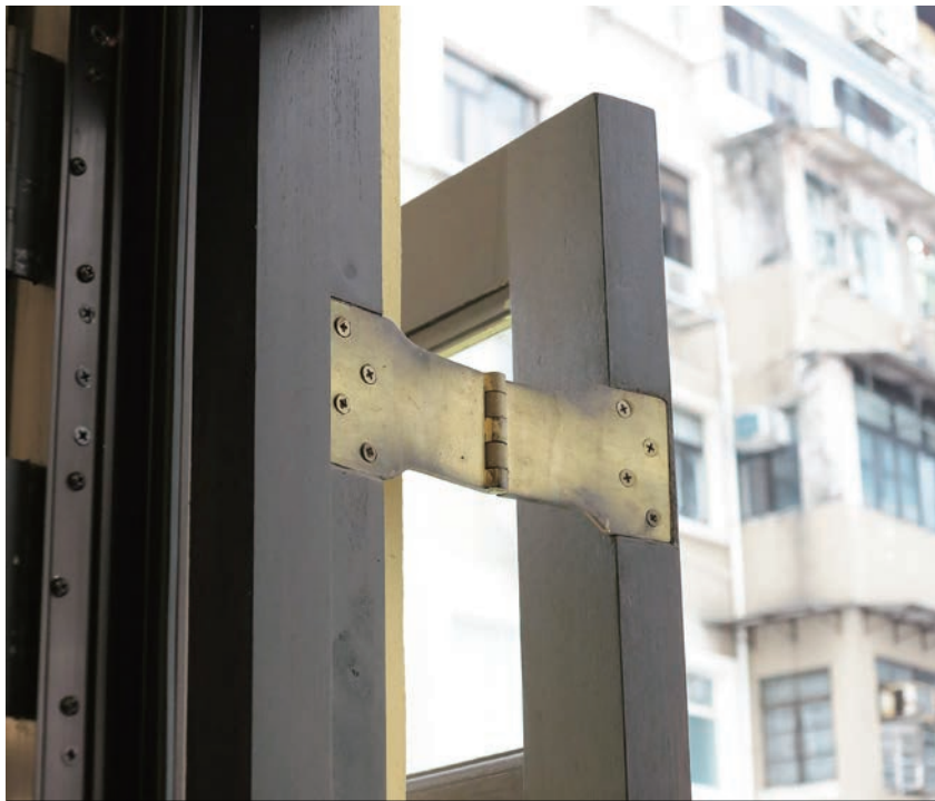
為求保留古蹟原貌，小至門鉸也一絲不苟。蘇彰德指，此“蝴蝶鉸”香港今已難覓，只能到內地訂造。 To preserve the original charm of the historical building, painstaking attention is paid to even the smallest details, such as door hinges. According to So, it is impossible to get this “butterfly hinge” in Hong Kong nowadays. It has to be custom-made on the Mainland.
